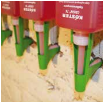
1 Horizontal barrier KÖSTER Crisin 76 Concentrate
