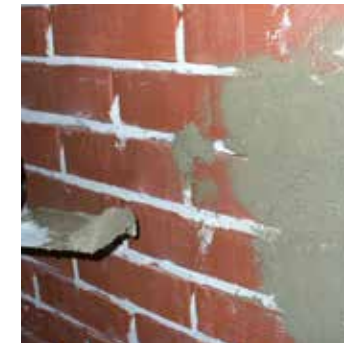
3 Repair and touch-up KÖSTER WP Mortar
