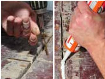
1. Substrate preparation: fastening of loose boards and sealing surface defects
