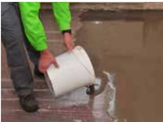
4. Distribute the material in the desired layer thickness directly after mixing (min. three minutes)
